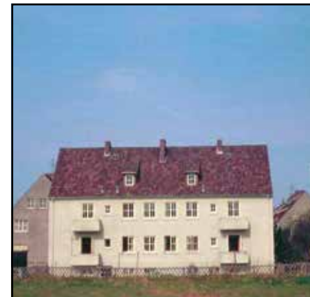
We were fortunate to live in the whole ground floor of this block at 8 Raabestrasse on the north-east fringe of the Stadt Park.
